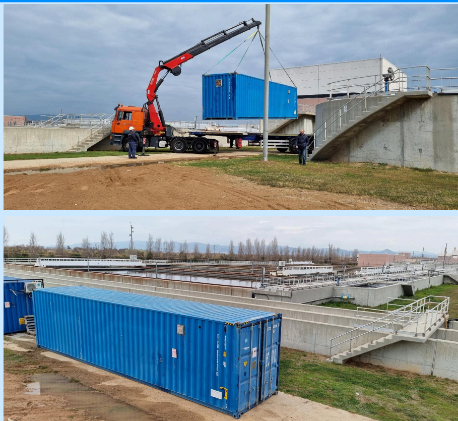
Figure 3. Downloading and installation of the BES container
