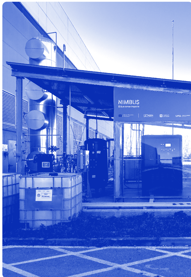
Image 2. General view of the LIFE NIMBUS pilot site.
